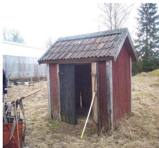
Spruthuset innan renovering.
