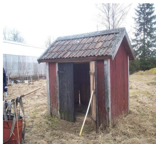
Spruthuset innan renovering.
